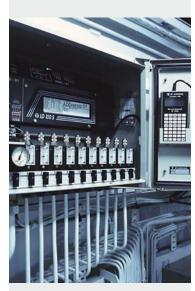
LevelDatic 100S cabinet with measuring air pipes on ship
